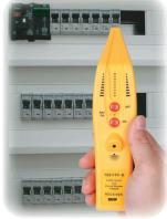
The circuit breaker that supplies the Transmitter circuitry is the one, that illuminates the greatest number of LEDs on the bar-graph and has the fastest buzz.
